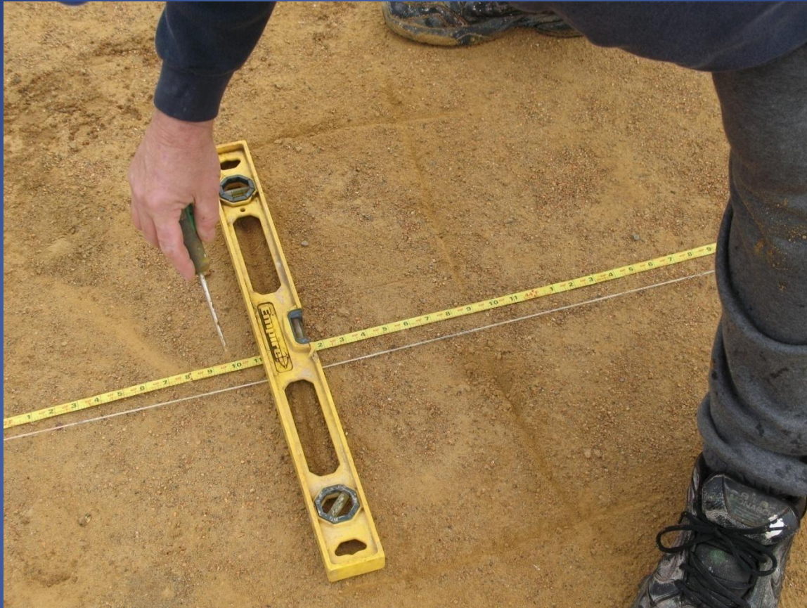
Marked Area to be Dug
